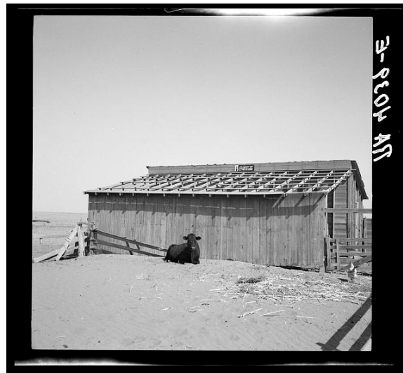
Figure 1 Image from the FSA collection and held by the LOC. Title: “This farmer took the roof off his barn to make a windbreak for his garden. There was no rain. Cimarron County, Oklahoma.” Photographer: Arthur Rothstein. Date Created: 1936.
